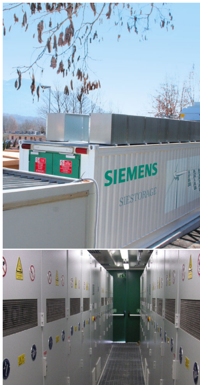
Fig. 2.8-8: SIESTORAGE has been installed with a performance of 1 MVA and a capacity of 500 kWh in the medium-voltage distribution system of Enel, the biggest power utility of Italy
